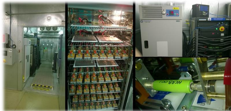
HNEI Battery lab
