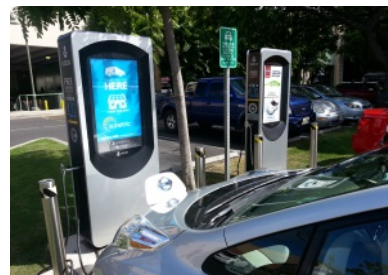
Figure 4. Hawaii Charging Stations (photo K. McKenzie)
